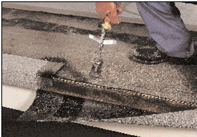
Folding and forming the well (1)
