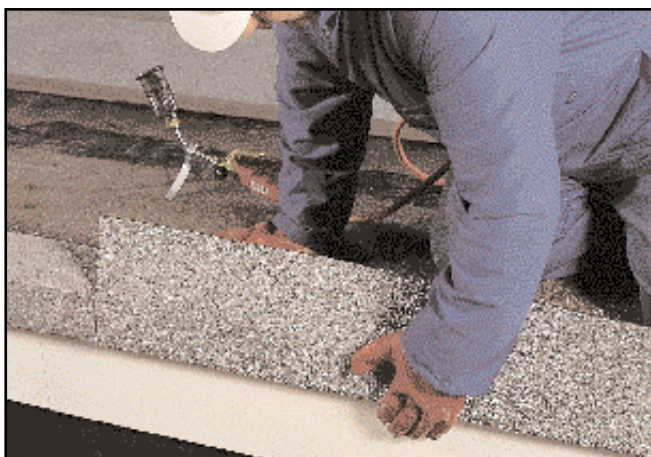
Folding and forming the well (2)
