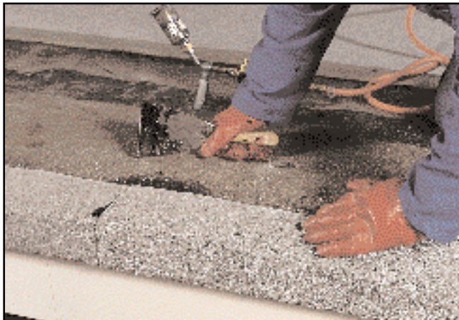
Folding and forming the well (3)
