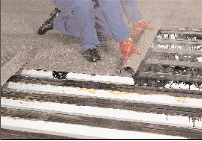
Application of vapour control layer to metal deck
