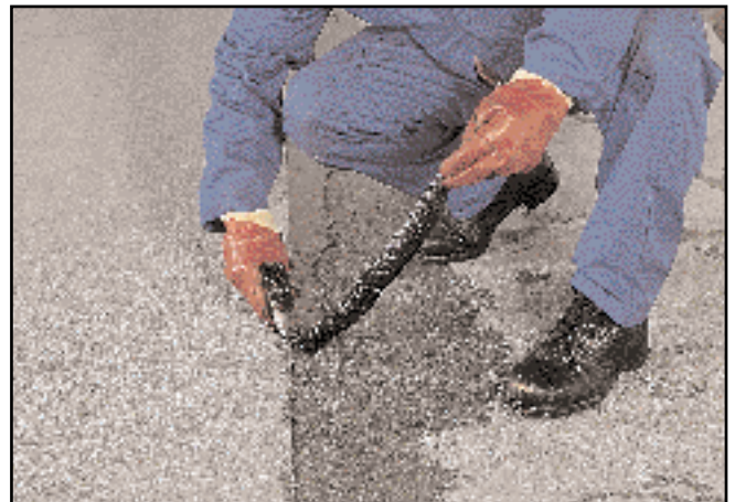
Wetting the edges and removing the excess bitumen
