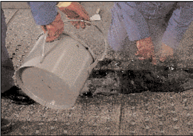
Application with type 3G to give a partial bond
