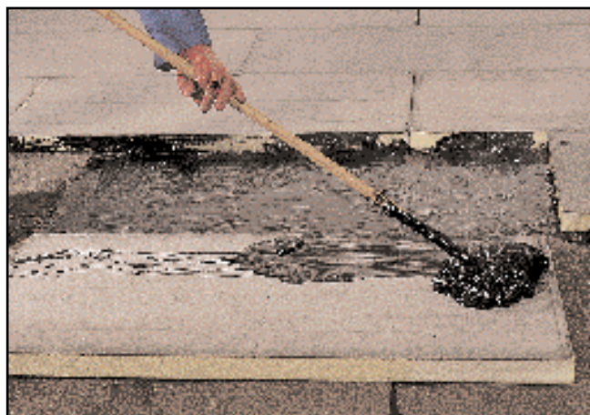
Application of insulation board
