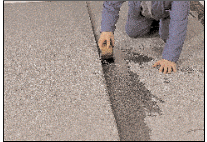
Wetting the edges and removing the excess bitumen
