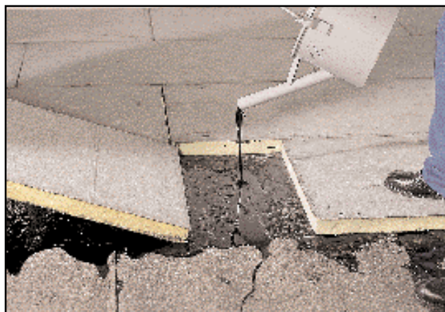
Application of insulation board
