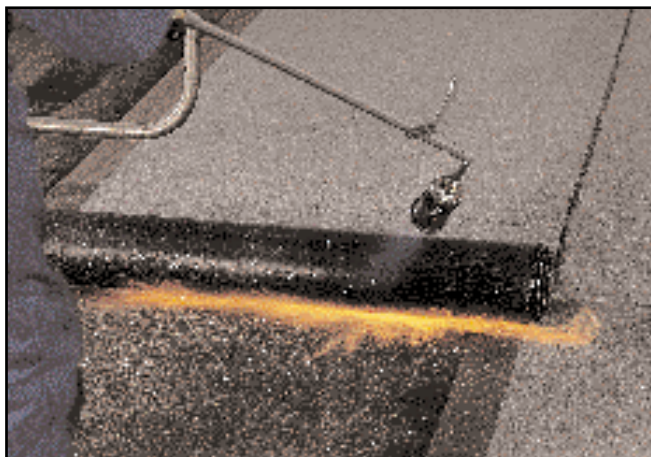
Torch application; note the bead of bitumen at the lap
